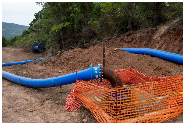
Figure 6 – Bypass installation phase
