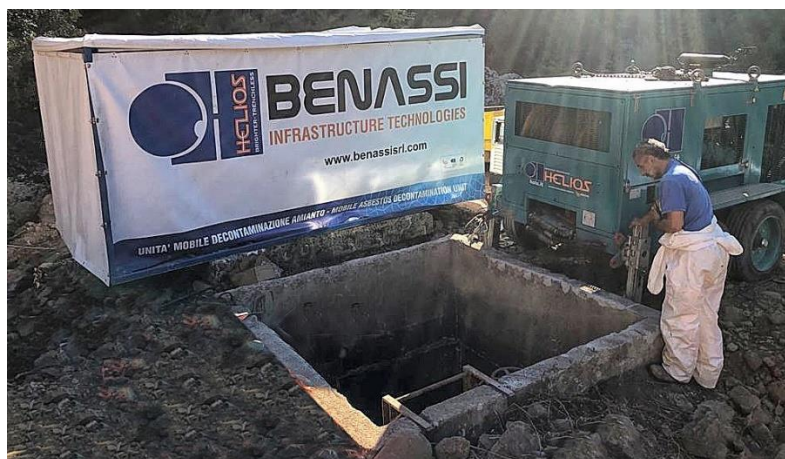
Figure 12 – Asbestos decontamination unit
