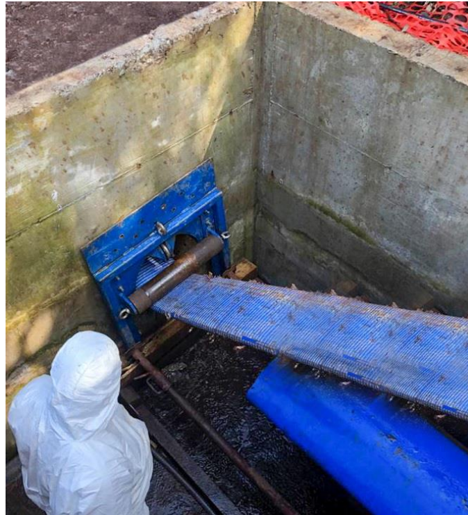
Figure 11 – Primus Line liner insertion
