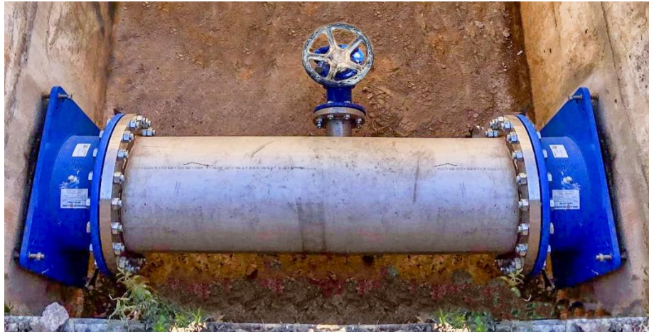
Figure 4 – Connectors customized for pits
