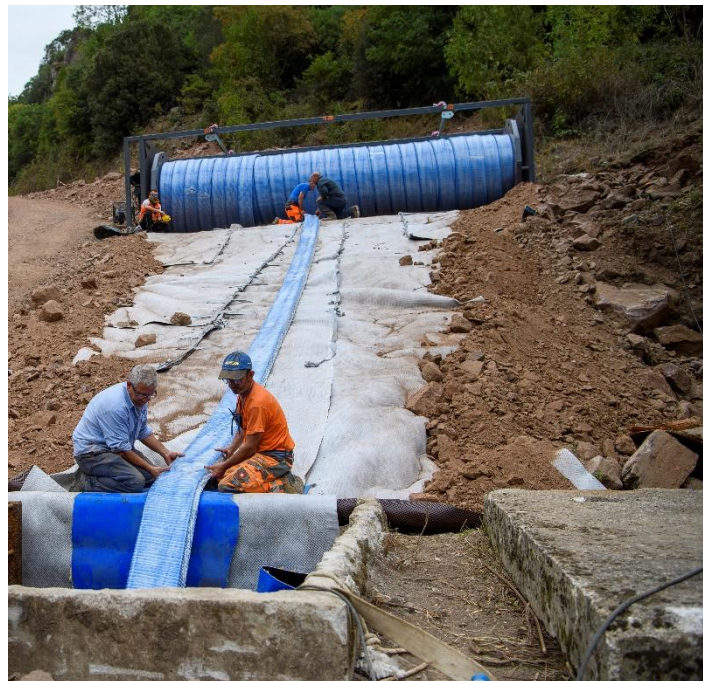
Figure 10 – Primus Line liner insertion
